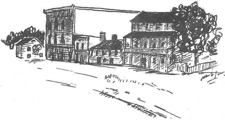
Sketch shows Fenton House and old tavern which stood on corner opposite the present Cambridge Grange Hall
